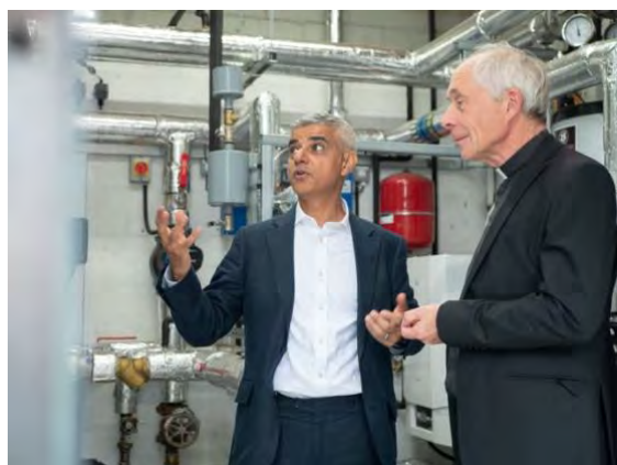
Sadiq Khan (left) Mayor of London inspects Air Source Heat Pumps
